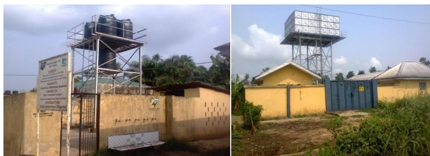
Plate 4.13: (1) Functional Water facilities at Agbia community; (2) Typical non-functional borehole at Ayama community and host of them in other communities.
