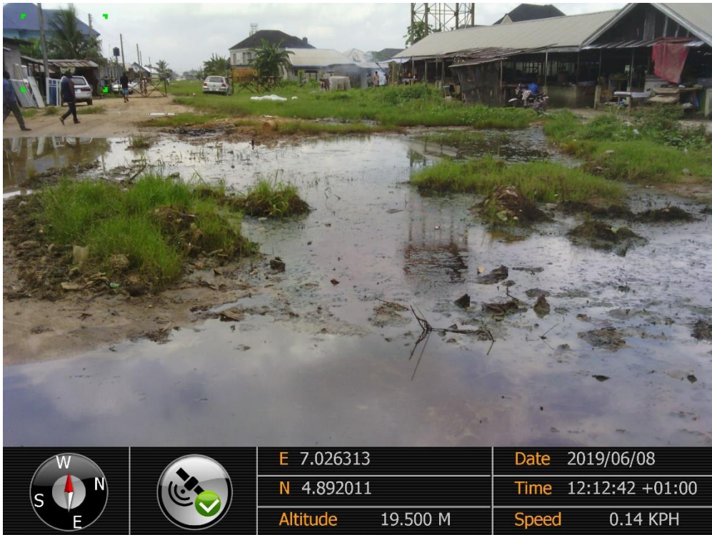
Overview: Part of spill impact on 28'' Nkpoku – Ogale Pipeline Right of Way at Rumuowha-Eneka. Picture was taken during Joint Investigation of 8 th June 2019.
