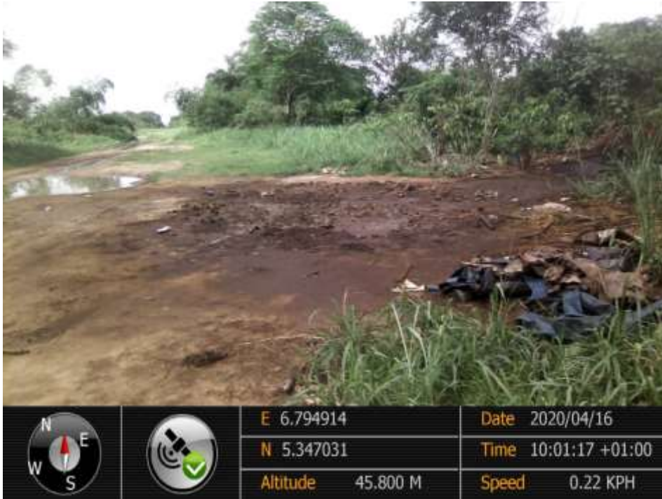
Overview: Part of spill impact on 18" Assa Rumuekpe Pipeline at Ochia. Picture was taken during Joint Investigation of 16 th April 2020.
