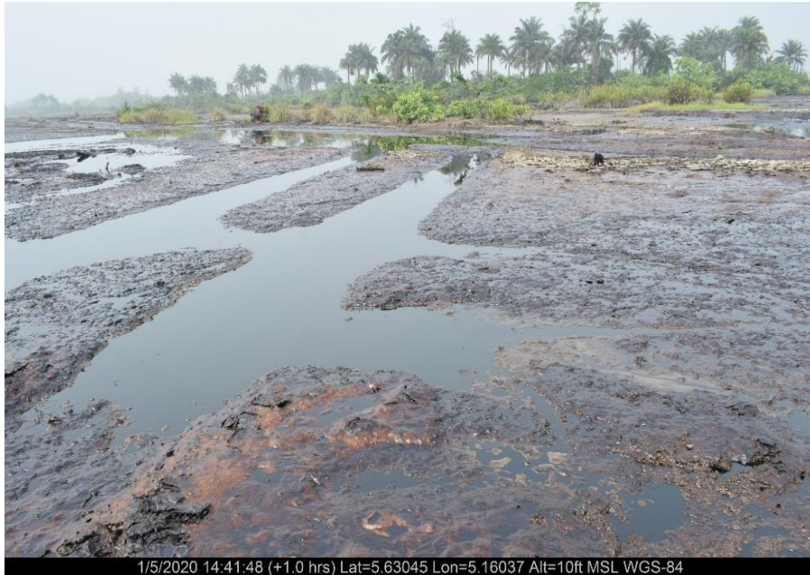
Overview: Part of spill impact on 20'' Trans Escravos Pipeline at Ugboegugun. Picture was taken during Joint Investigation of 5 th January 2020.
